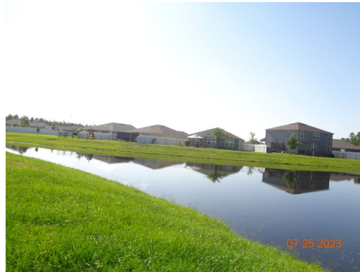
Pond 11: Previous treatment was effective.
